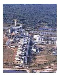
In the Smelter the process consists of the Electrode and Potroom areas and the Ingot Plant. In the potrooms the electrolytic dissociation of alumina, dissolved in a molten electrolytic bath by means of direct electric current, is performed. This process, carried out in pots operating about 950°C, results in molten aluminum, which is transported in crucibles to the ingot plant.
