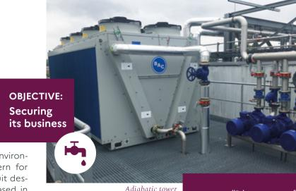
technology) to provide a closed circuit for the refinery condenser cooling network resulting in savings of 76,000 m<sup>3</sup>/year (equivalent to more than 20 Olympic-size swimming pools).
