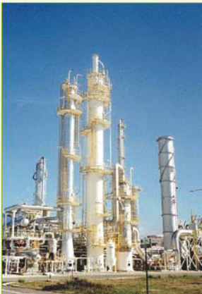
CO 2 post-combustion capture at a plant in Malaysia. Courtesy of Petronas Fertilizer Kedah and Mitsubishi Heavy Industries.
