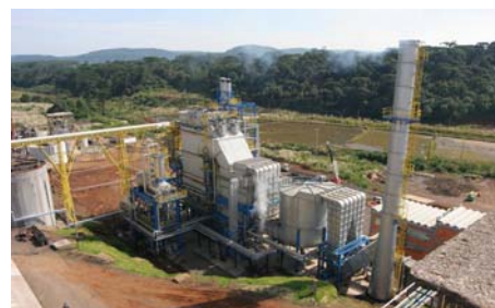
The new Irani biomass facility.
